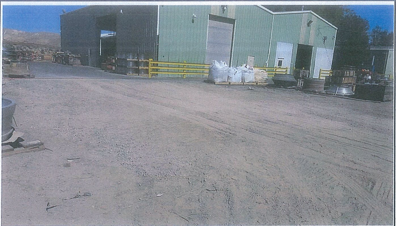
Photo 7: Area 1 following backfill, compaction, and grading, looking east-southeast.
