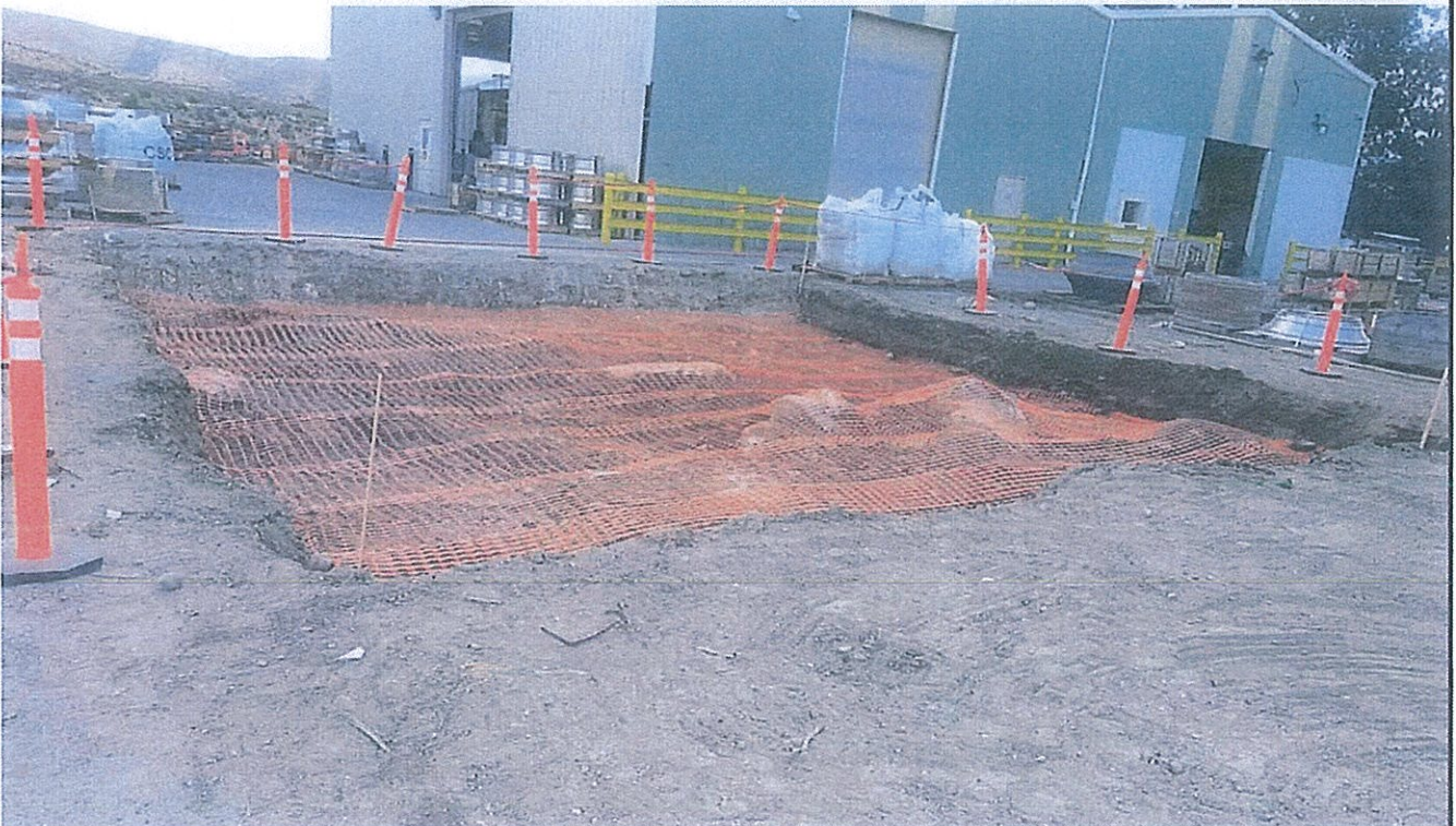
Photo 6: Area 1 prior to backfilling.
