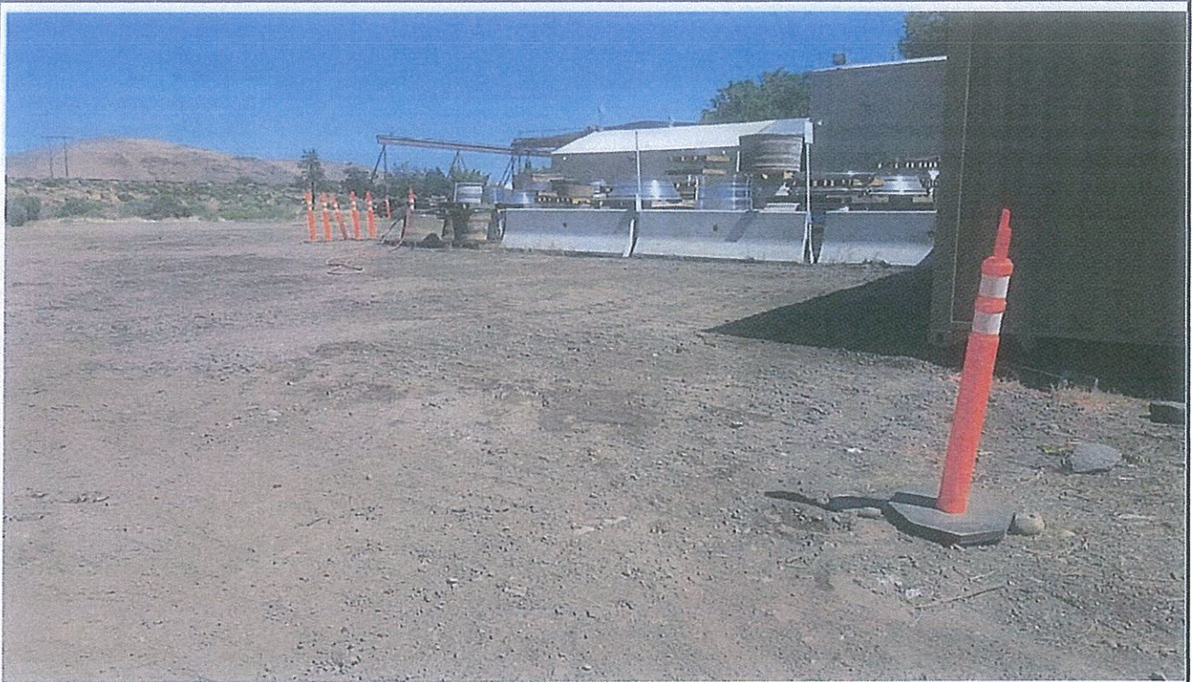
Photo 9: Area 2 following backfill, compaction, and grading, looking east.
