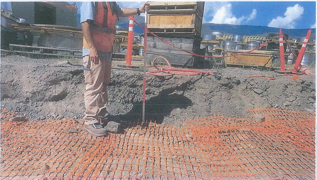
Photo 12: Confirmation of excavation depth in Area 3.
