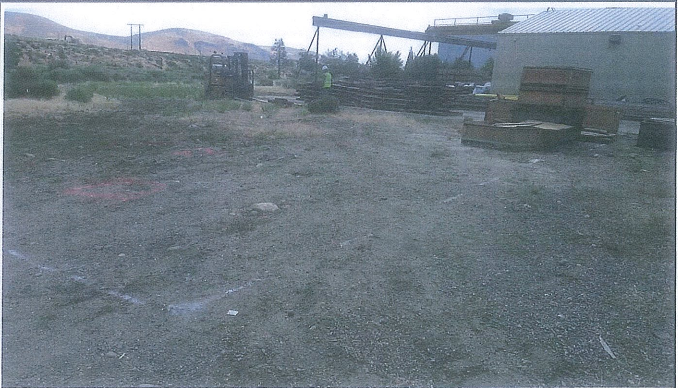
Photo 1: Markout of excavation areas; Area 2 shown.
