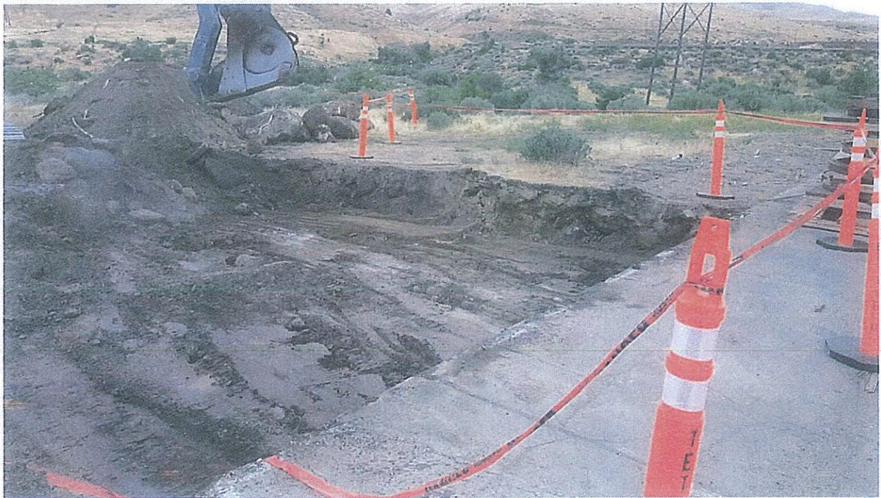
Photo 10: Excavation in progress on Area 3.
