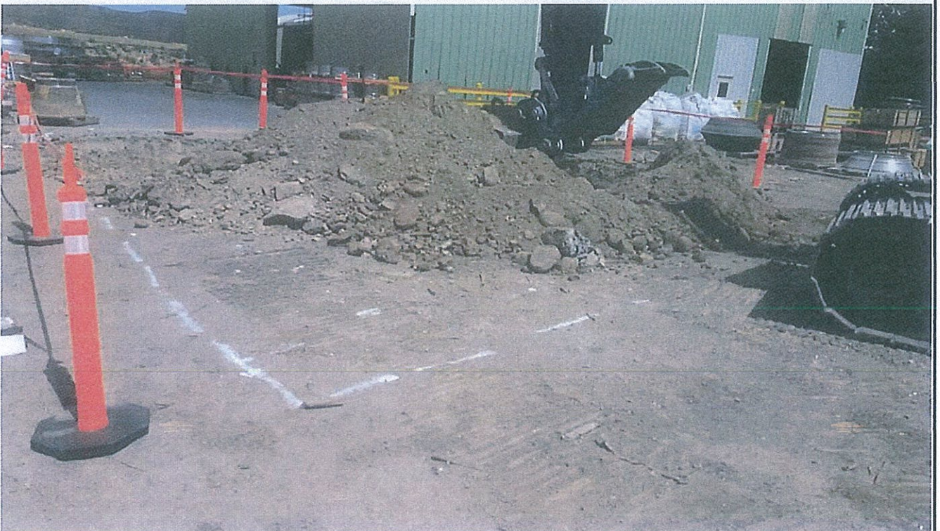
Photo 2: Starting excavation of Area 1.
