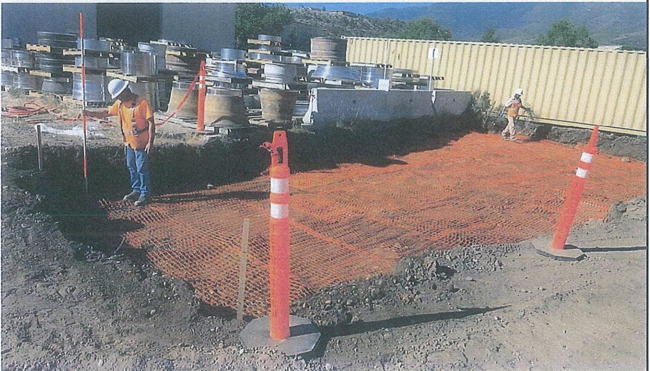
Photo 8: Area 2 prior to backfilling.
