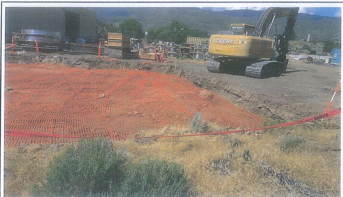
Photo 13: Area 3 excavation ready for backfill.
