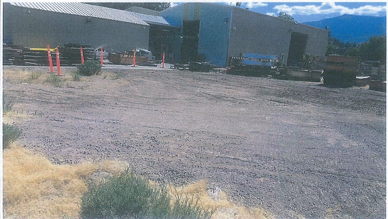
Photo 14: Area 3 following backfill, compaction, and grading, looking south-southwest.
