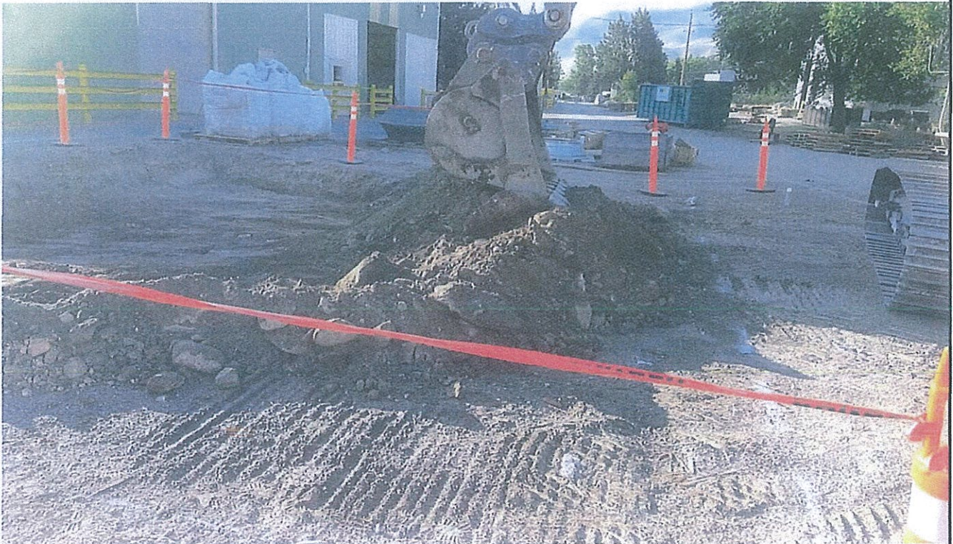
Photo 4: Area 1 excavation progressing.
