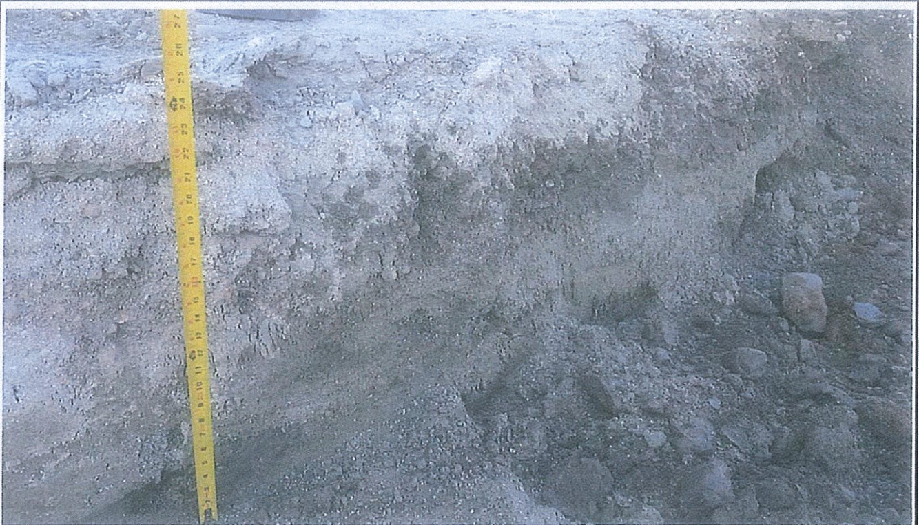
Photo 5: Checking depth of the excavation.
