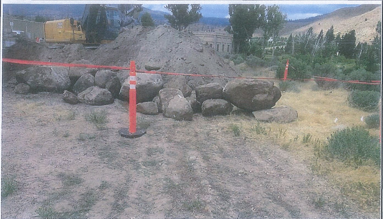
Photo 11: Boulders removed from the excavation and set aside; these boulders were returned to the excavation, as possible.
