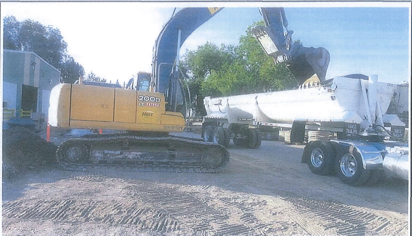
Photo 3: Loading soils into trucks for transport to the landfill.
